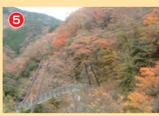
Sendan Todoru Suspension Bridge
